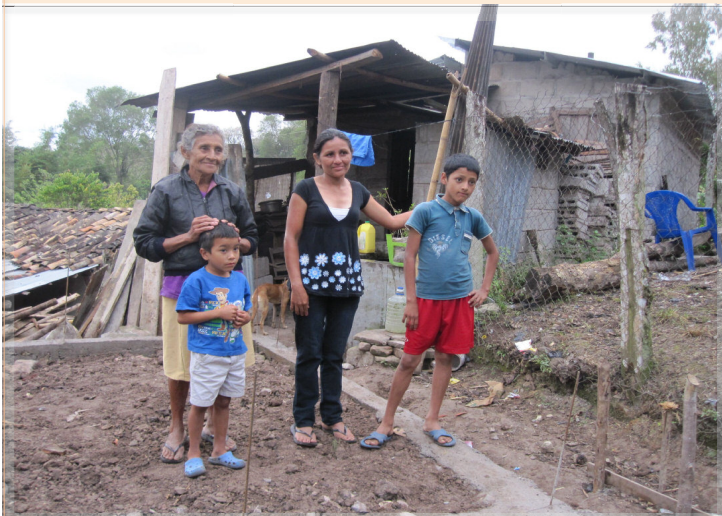
A family in Trinidad de Copan stands by the foundation of their new home being built with the assistance of the village and volunteers.
